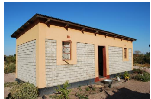
Figure 1: House built from SSBs.
